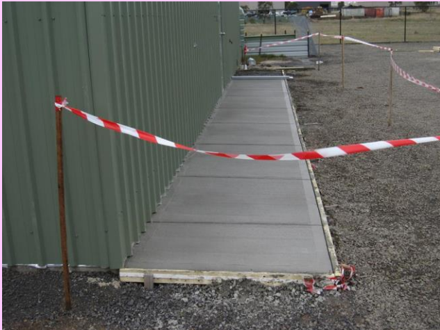
Freshly laid concrete path
