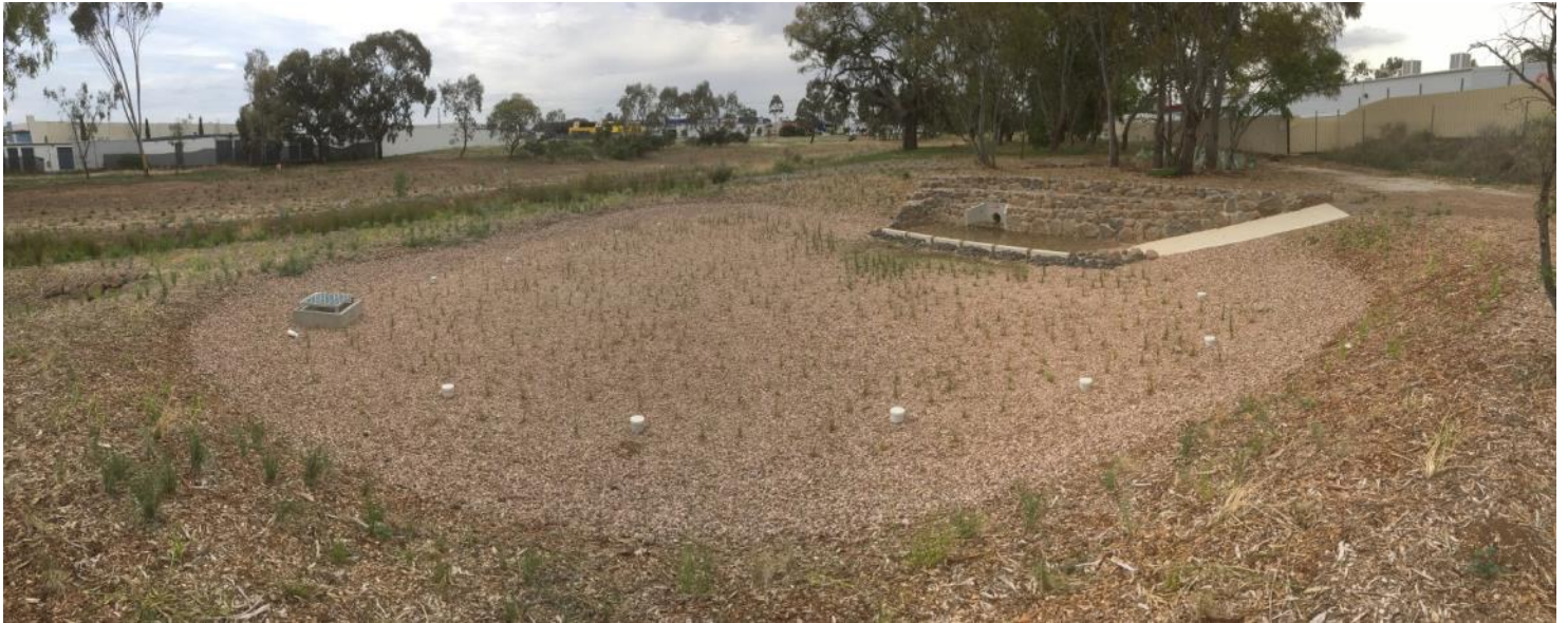
New Rain Garden - Ryans Creek North
